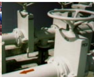
Fully closed, the Series 75 ensures drop-tight, bi-directional shutoff and an intrinsically safe design with no packing to maintain.
