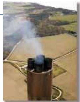
*Blue and white smoke is evidence of SO<sub>3</sub> present in the stack gas as condensed sulphuric acid. Monitoring of opacity (whilst useful) will not reveal the underlying problem.*
