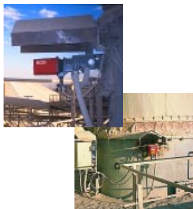
Dust monitoring on a cement plant
