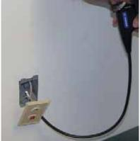
Inspect electrical wire routing and condition or HVAC ducts for leaks and dust buildup.
