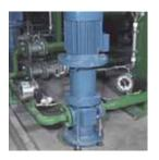
Pump: KF 20 to KF 550. Medium: Polyol, isocyanate. Delivery rate: 282 I/min. Speed: 750 min<sup>-1</sup>. Pressure: 10 bar. Temperature: Ambient. Viscosity: Polyol to 5.000 mm<sup>2</sup>/s, isocyanate
